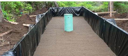
Liner installation
