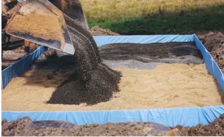
Filter sand and distribution bed
