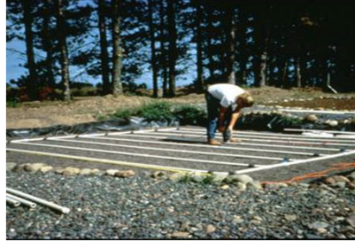
Drilling manifold 'orifices'
