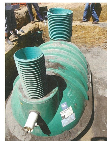
Figure 6. Installation of a STEP tank.
