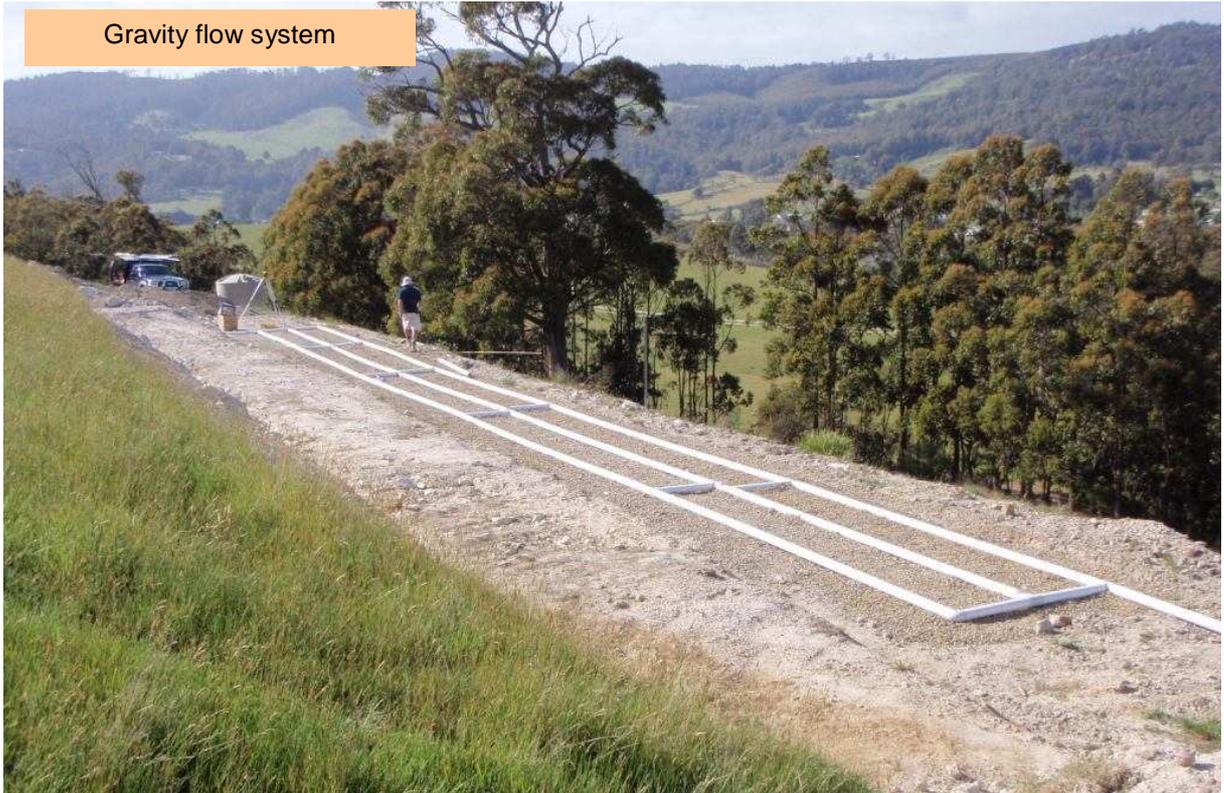
**Above.** This nonconventional bed received gravity flow wastewater from a septic tank up the slope at right.
