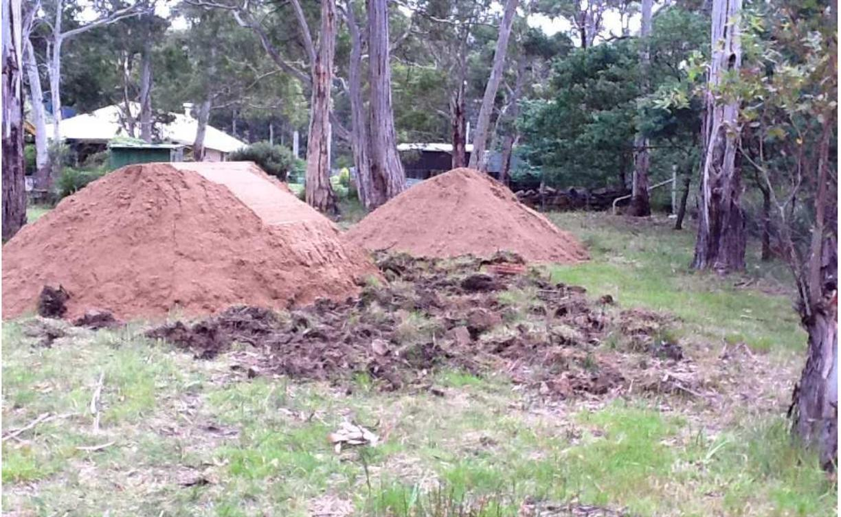
Plate 1 (above). Rip beneath basic module; stockpile filter sand. The soil is Category 6 clay to the surface. The PDA is sized to account for this, using a DLR of 3mm/day.
