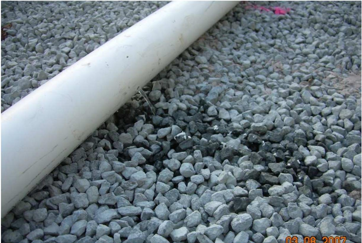
Plate 5 (above). Perforated pipework under test.
