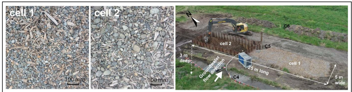
Fig. 3. Pictures of the 50/50 woodchip/gravel mixtures that make up the denitrification wall, and a photo showing installation works. Cell 1: chipped wood mixed with 20–40 mm gravel rounds. Cell 2: hogged wood mixed with parent aquifer material, screened of material under 20 mm diameter. The positions of monitoring wells C4:C6 are marked on the photo.
