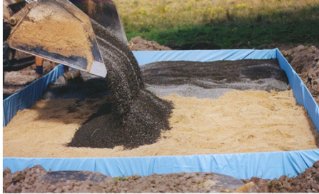
Filter sand and distribution bed
