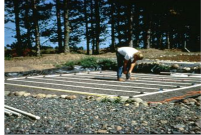
Drilling manifold 'orifices'
