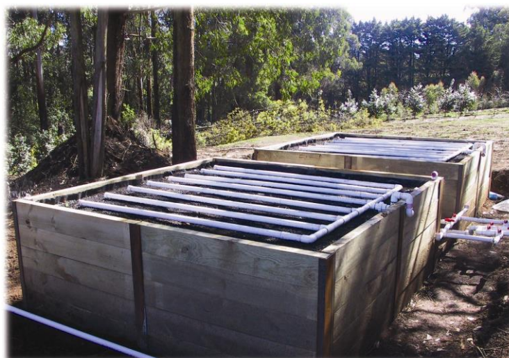
Figure 2. View of the two biofilter boxes, showing the removable distribution manifolds and the transfer / linking / isolation pipework (at right, between the units)
