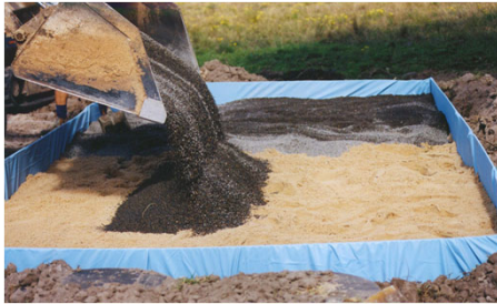
Filter sand and distribution bed
