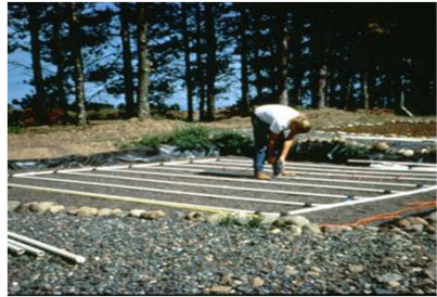
Drilling manifold 'orifices'
