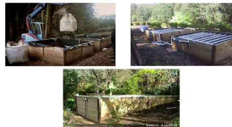
Peat Biofilter installation, VIC
