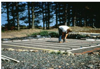
Drilling manifold 'orifices'
