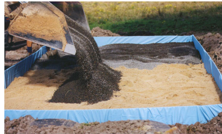
Filter sand and distribution bed
