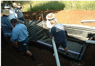
Underdrain and gravel bed
