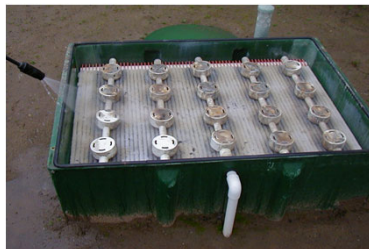
Orenco Advantex fabric filter
