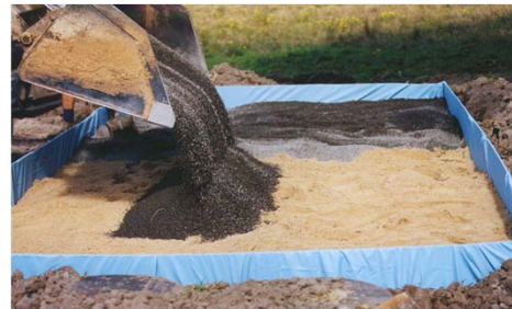
Filter sand and distribution bed
