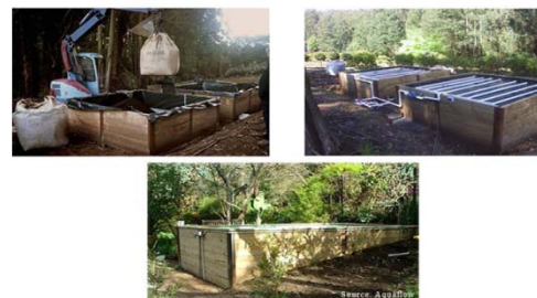
Peat Biofilter installation, VIC
