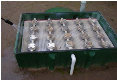
Orenco Advantex fabric filter
