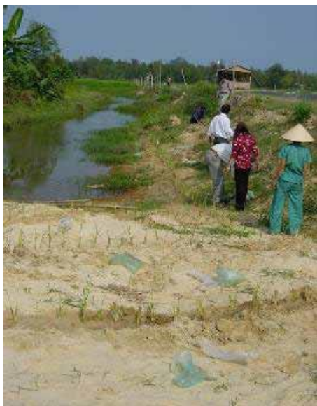
Photo 8: Left: March 2002: VS trial at the edge of a shrimp pond, where a canal drains flood water to Vinh Dien River; right: November 2002: mass planting combined with rock riprap to protect bank along Vinh Dien river
