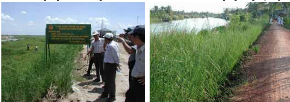
Photo 15: In An Giang Vetiver stabilizes a river dike (left), and a natural river bank (right)
