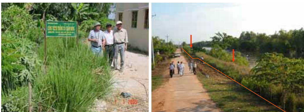
Photo 16: Left: Vetiver borders the edge of flood resettlement centres; right: the red markers delineate about 5 m (15') of dry land saved by Vetiver
