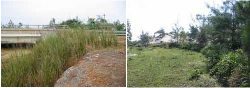
Photo 6: Left: Vetiver protects bridge abutment along Nat. Highway nr.1; right: December 2004, local species have replaced Vetiver
