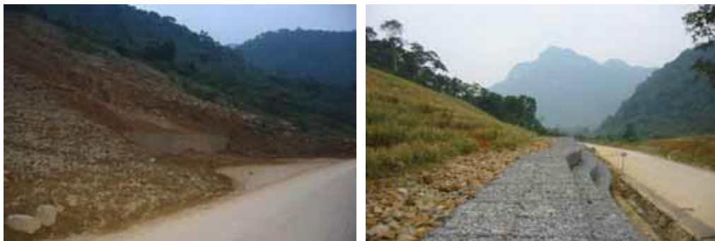
Photo 21: Da Deo Pass, Quang Binh: Left: Vegetation cover is destroyed, revealing ugly and continuous failures of cut slopes; right: Vetiver rows on top of the slope very slowly squeeze down, considerably reducing the failed mass
