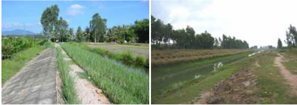
Photo 12: Upstream anti-salinity dike section with traditional concrete riprap facing the river (left) and along a section of the irrigation canal, surface erosion mars the opposite bank (right)
