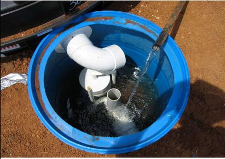
Greywater septic tank to dosing chamber, near Nimbin, NSW
