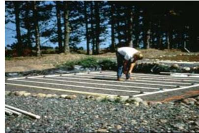
Drilling manifold 'orifices'
