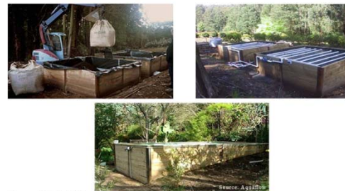
Peat Biofilter installation, VIC
