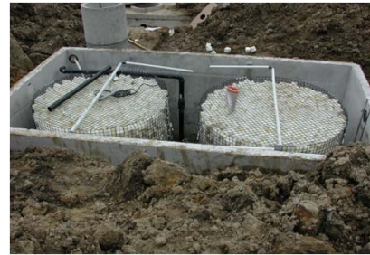
Waterloo Biofilter, Canada
