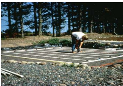
Drilling orifices
