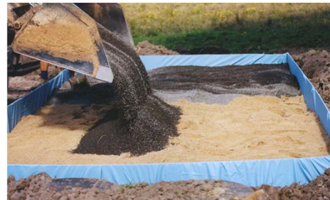
Filter sand and distribution bed
