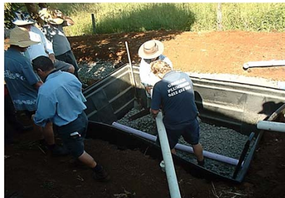
Underdrain and gravel bed
